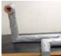
Heated transfer lines
